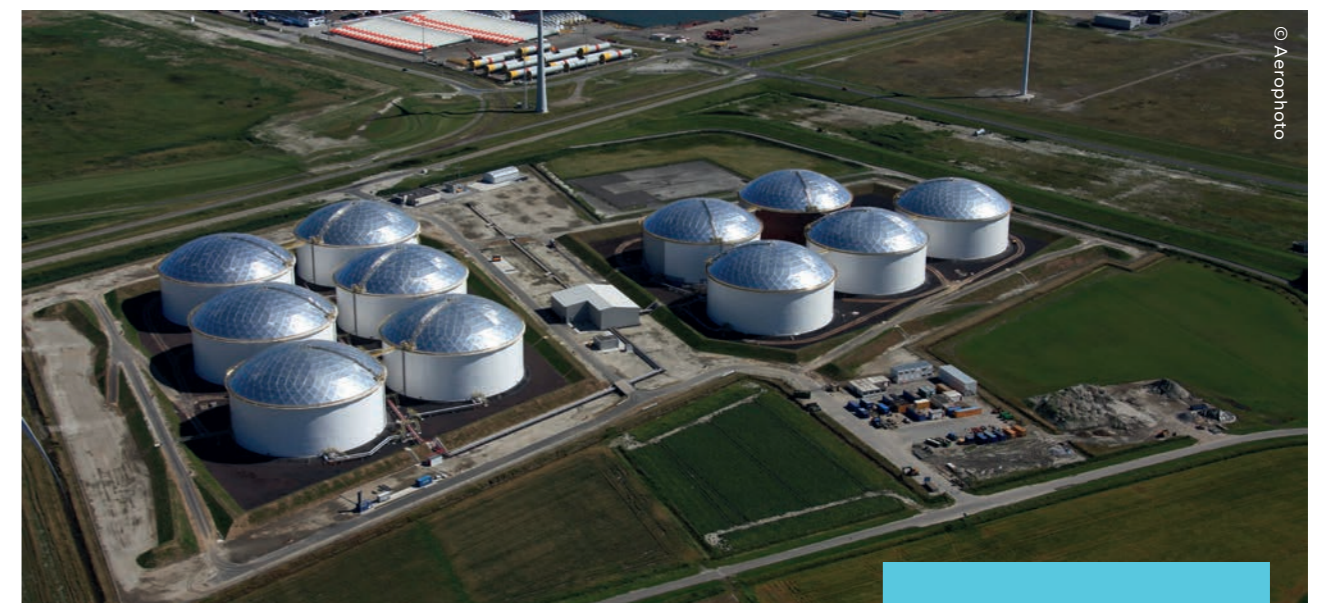
Vopak-Tanklager in Eemshaven
